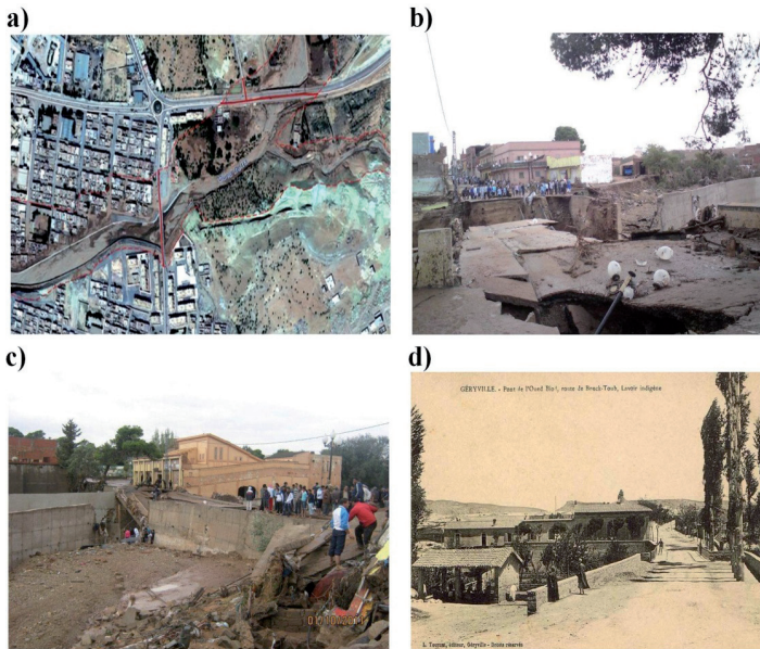
Figure 3. Impact of flooding – El Bayadh City on October 01, 2011. a) Satellite images, Algerian Alsat-2A [ASAL, 2011], b), c) and d) Destruction of the Historical Mahboula Bridge.
